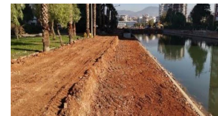
IAC7 – Culvert works on Peynircioğlu stream along 1.6 km
