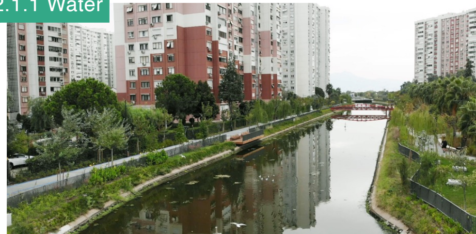
Figure 2.1. Culvert works for Peynircioğlu River – İzmir (Turkey)
