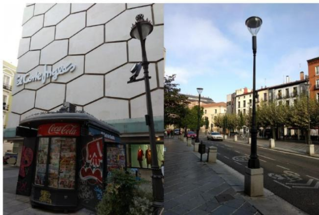
Figure 4.1: Mobile Air quality sensors installed close to the Green façade in Valladolid (CARTIF)
