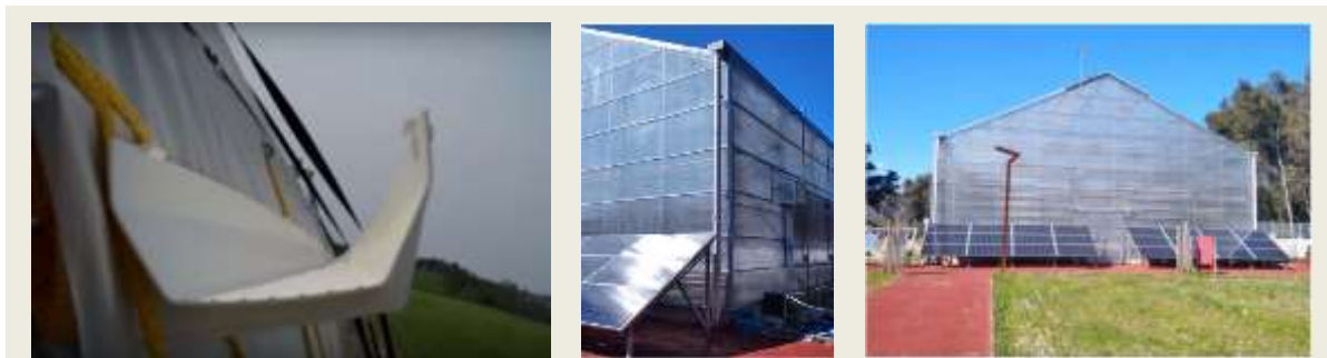
Figure 1: Collecting and transferring rainwater from the roof of the greenhouse to the tank
