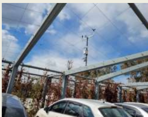
Figure 6: Fixed station at Vilayetler Evi Parking Lot (March 2022)
