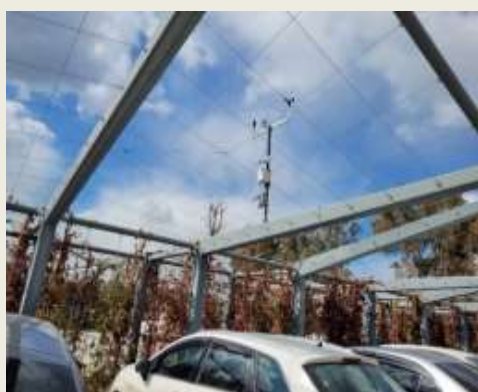
Figure 6: Fixed station at Vilayetler Evi Parking Lot (March 2022)
