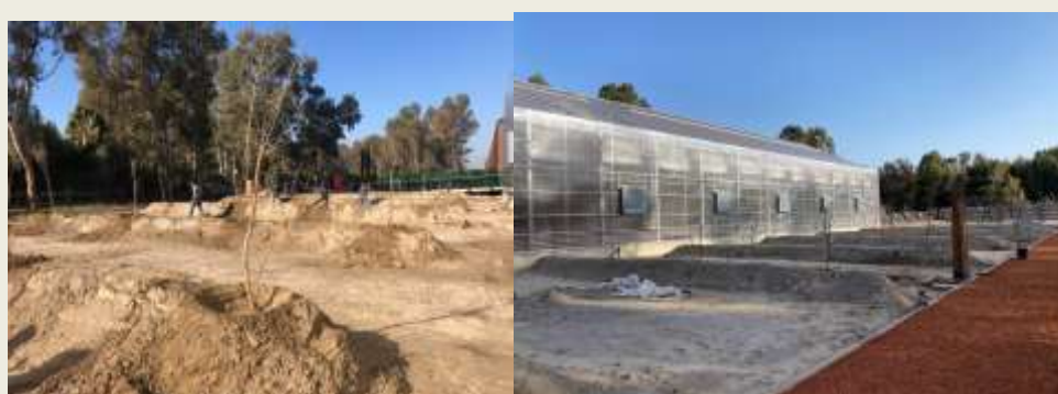
High ridge type soil pads on salty ground and fruits plantation
