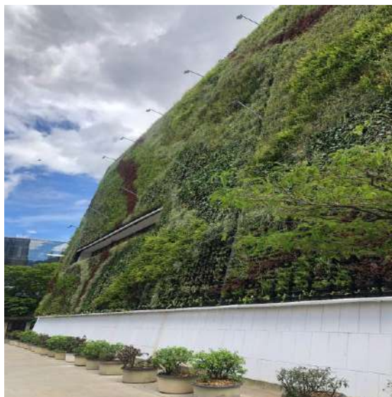
Figure 4.31: Example of a green wall in Medellín
