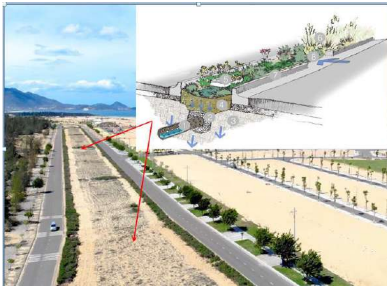
Figure 5.48: Rain garden on the median strip of Nhon Hoi economic zone traffic route
