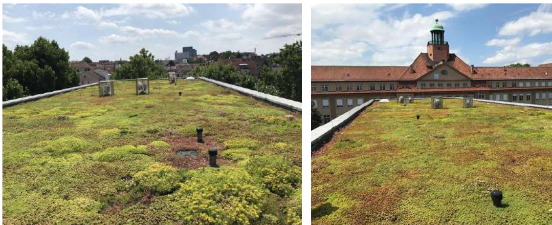
Figure 2.24: Green roof on a municipal building
