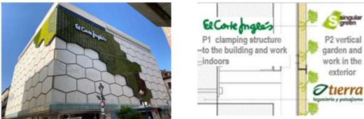
Figure 3.5: Public-Private agreement for the Green Façade in Valladolid
