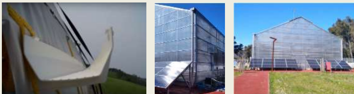
Figure 1: Collecting and transferring rainwater from the roof of the greenhouse to the tank
