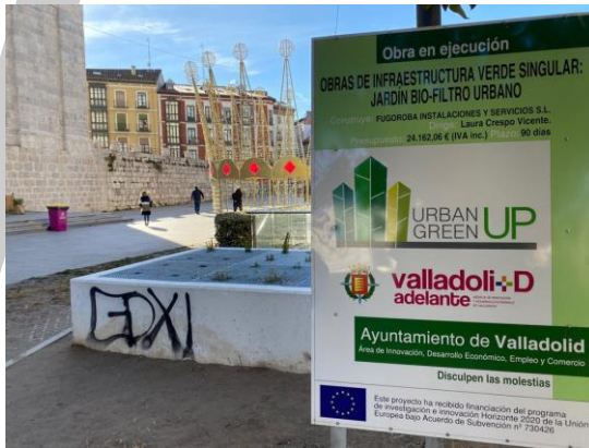
Vandalism (graffitti) (Dec 2021)
