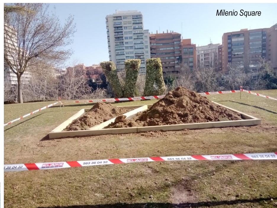
Construction of the Natural Pollinator's Modules in the Green corridor (Milenio Square) (VAc19)
