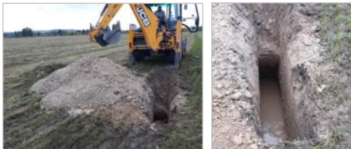
Figure 4.47: Excavator machine used to dig the pits and take out the terrain for its study (Source: Duero River Basin Authority).
