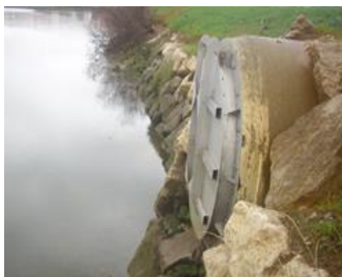
Figure 4.54: Detail of a non-return valve (Source: Duero River Basin Authority).
