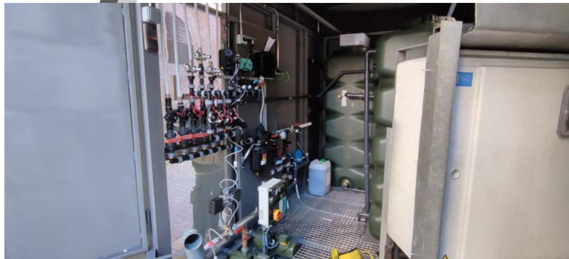
Green shady structures irrigation system: water recirculation with pumping system
