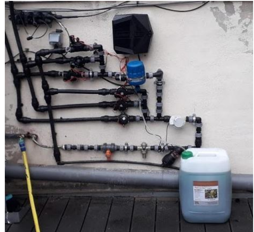
Green roof garden irrigation system
