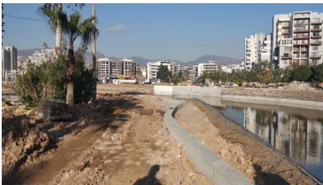
Figure 4-27: Concrete foundation of green fences
