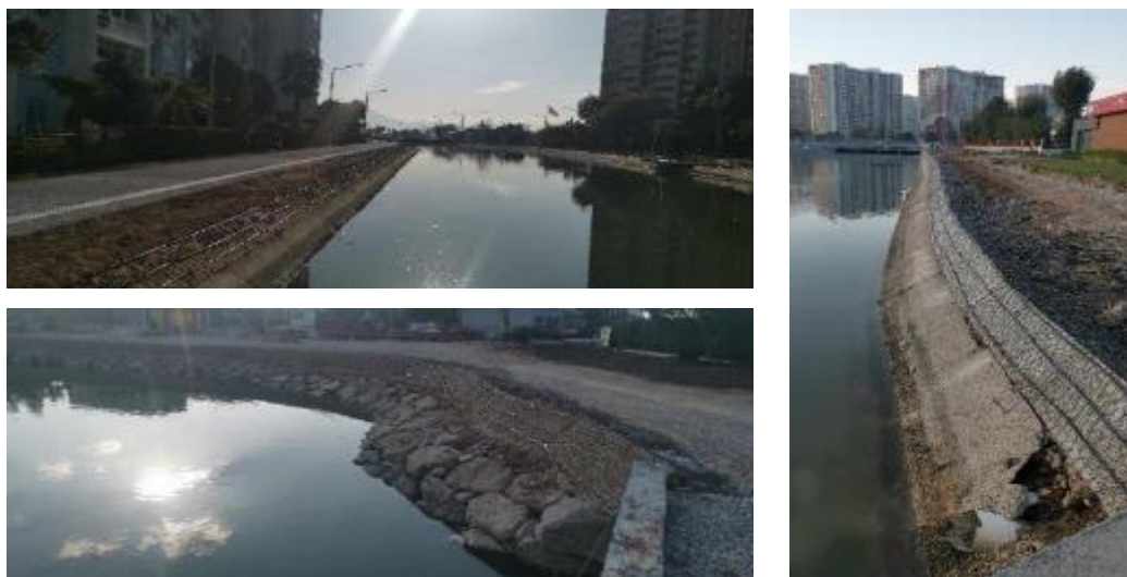
Figure 4-19: Completed implementation of terramesh system
