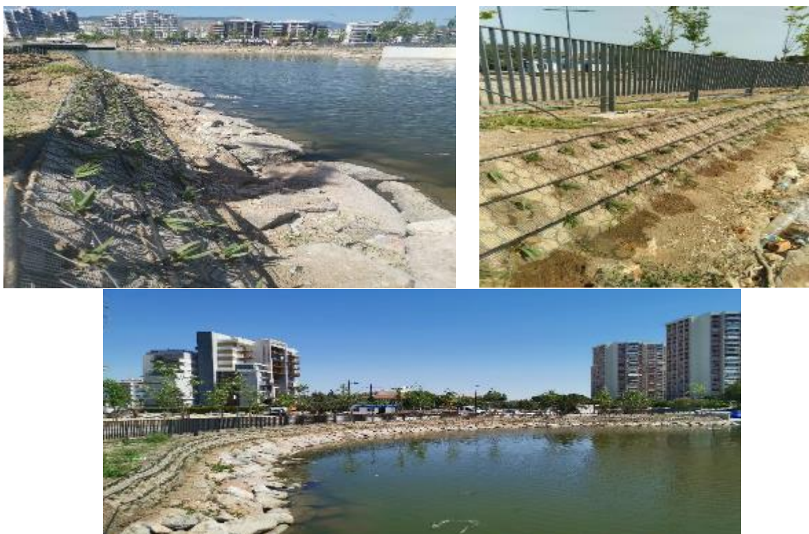
Figure 4-23: Final view from in-stream culvert works
