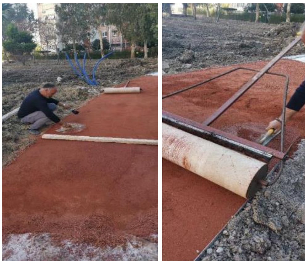
Figure 4-8: Tile dust laying
