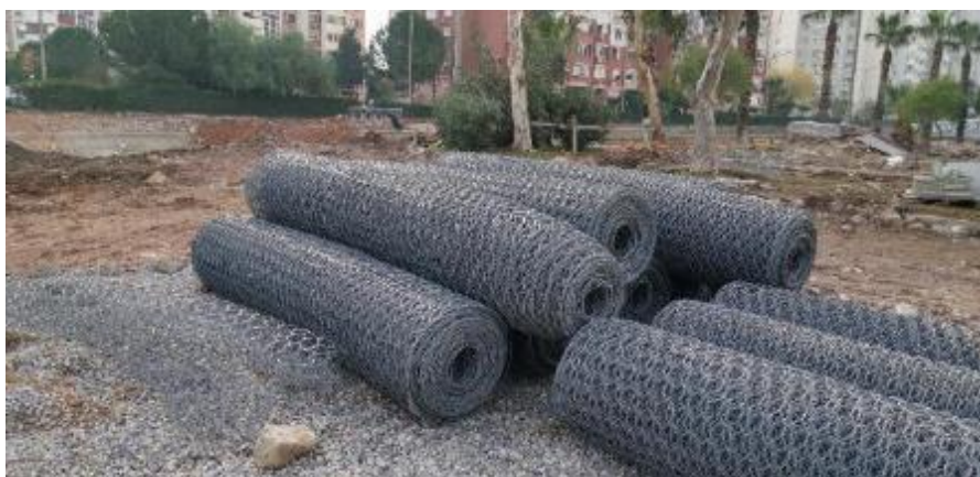
Figure 4-13: Terramesh materials on site
