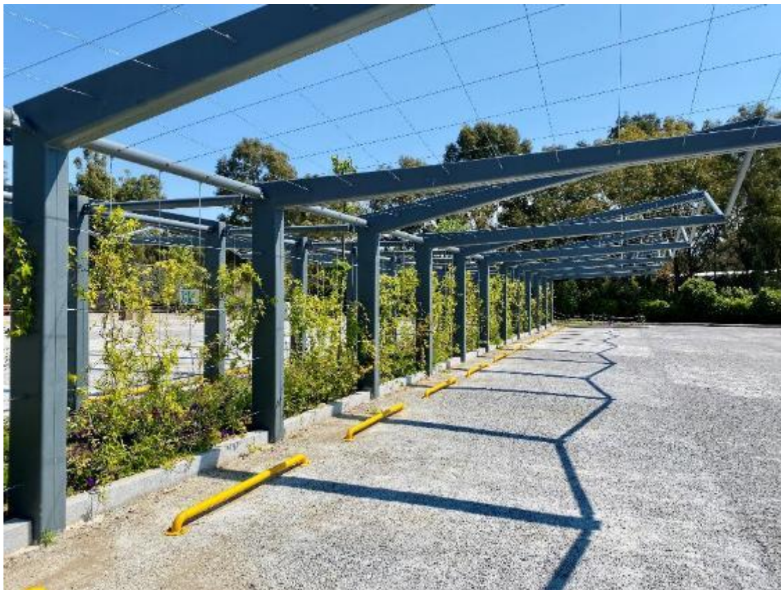
Figure 2-5: Final view of green covering shelter, permeable surface and ivy plants on biochar added soil
