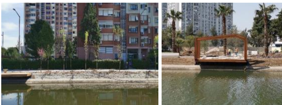
Figure 4-20: Implementation behind the terramesh area
