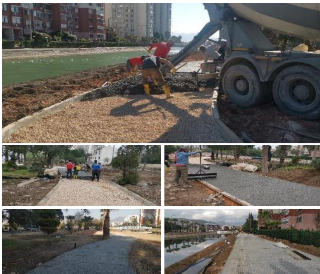
Figure 4-6: Pouring and levelling of permeable concrete
