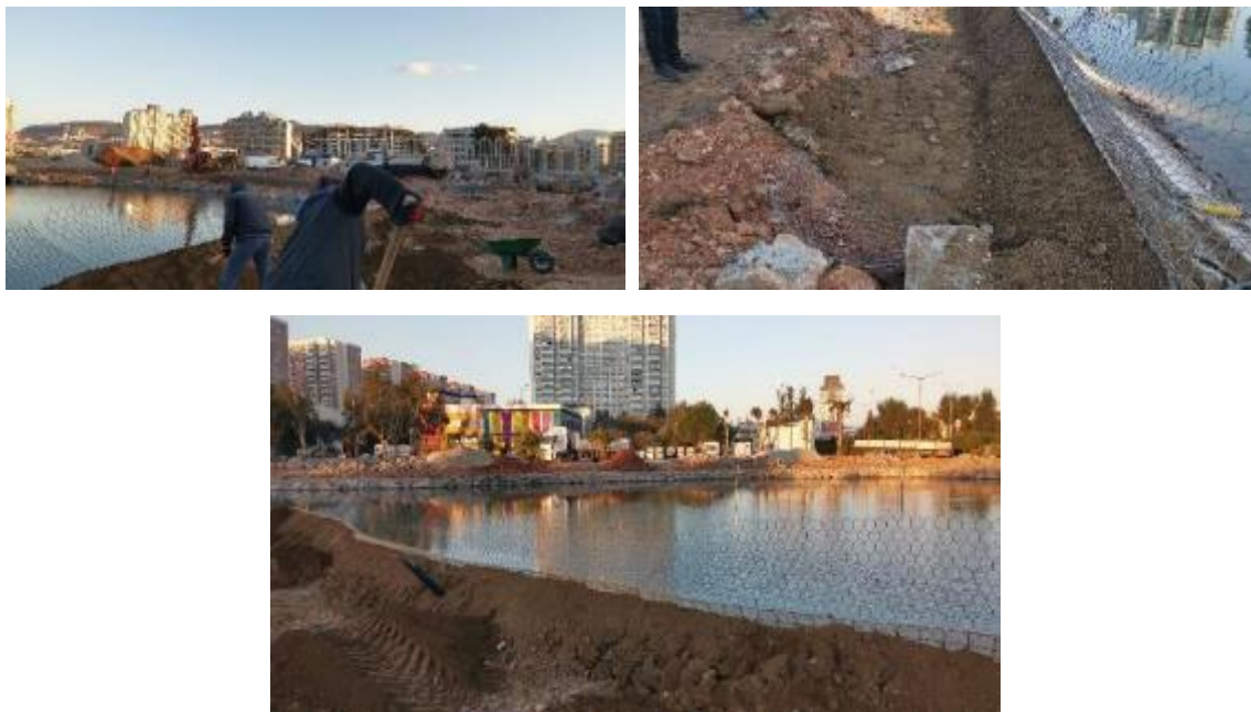
Figure 4-16: The area after pouring vegetation soil
