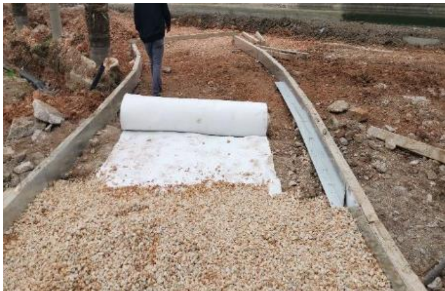
Figure 4-3: Geotextile layer laying
