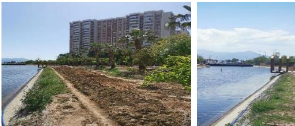
Figure 4-21: Terramesh area with plants
