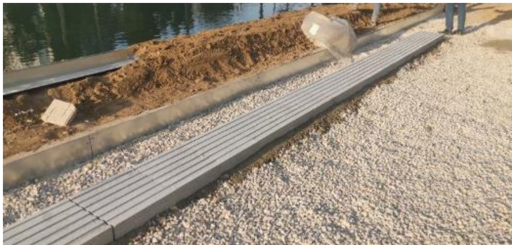
Figure 4-5: Channeled brick on filling layers
