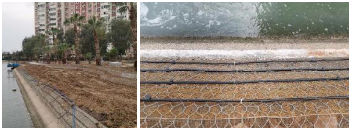
Figure 4-18: Implementation of drip irrigation system
