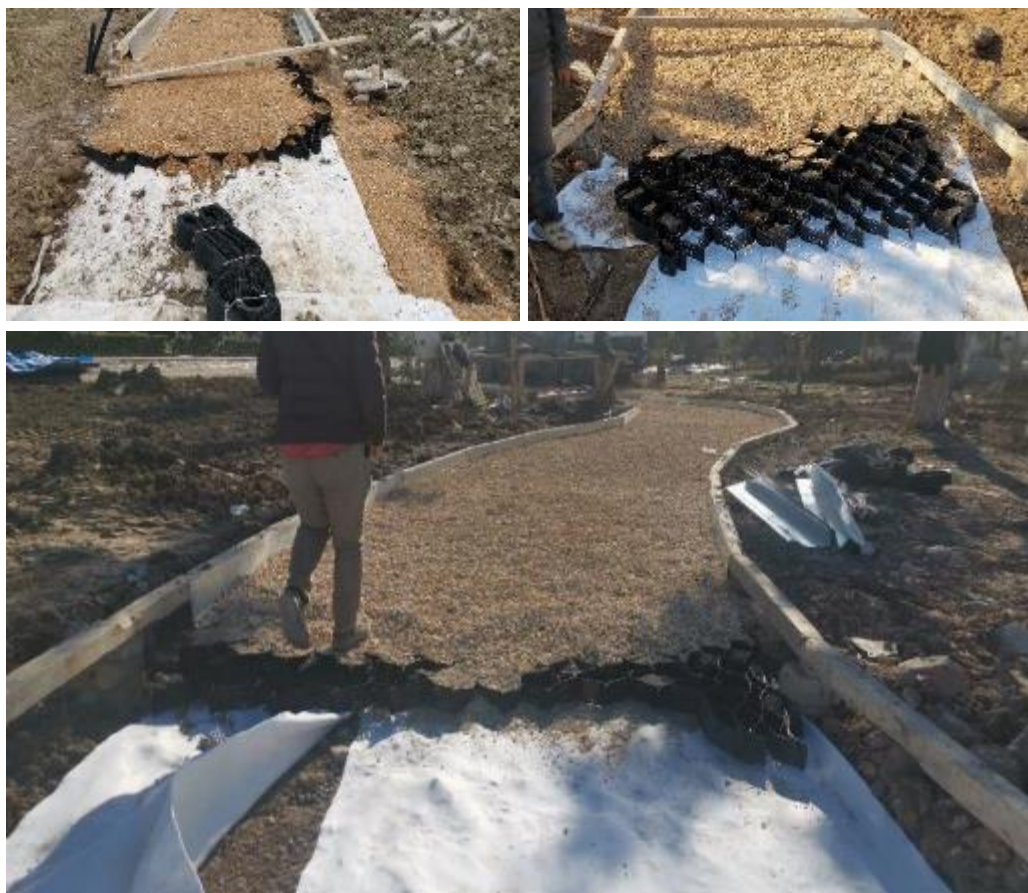
Figure 4-4: Cellular and granular filling operations
