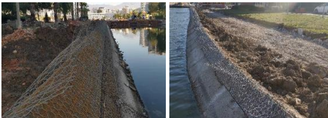
Figure 4-17: Implementation of terramesh layers
