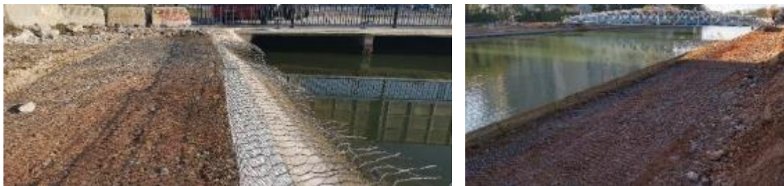
Figure 4-15: Terramesh material on excavated surface
