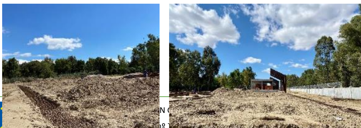
Figure 3-4: Reinforcement and ground preparations of climate-smart greenhouses
