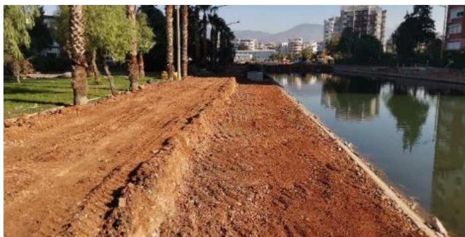
Figure 4-14: Area of terramesh application after excavation
