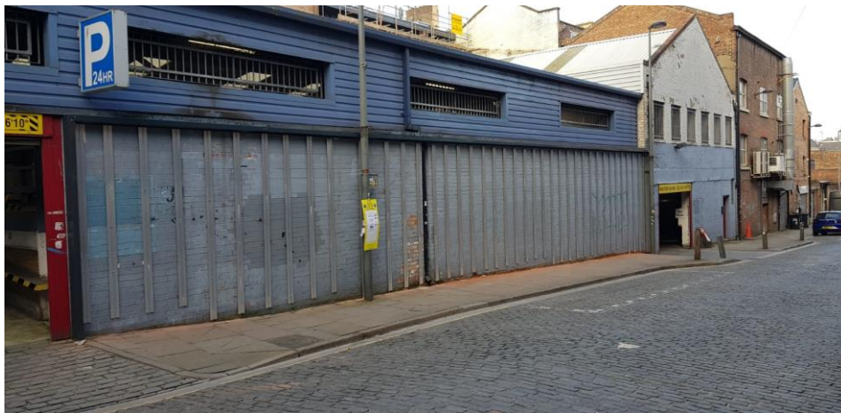
Figure 31: Green wall batons, preparation of site
