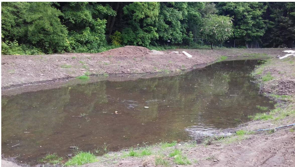
Figure 17: Main pond in place awaiting planting
