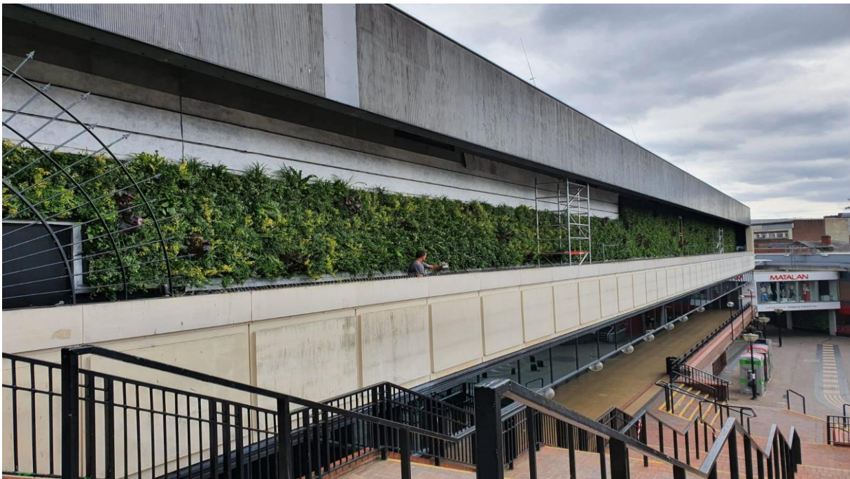
Figure 33: Works underway at Demo B green wall
