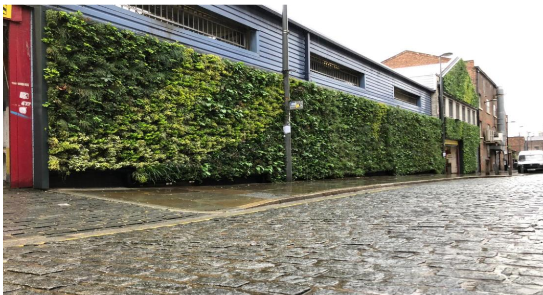
Figure 32: Completed green wall in place, Parr Street
