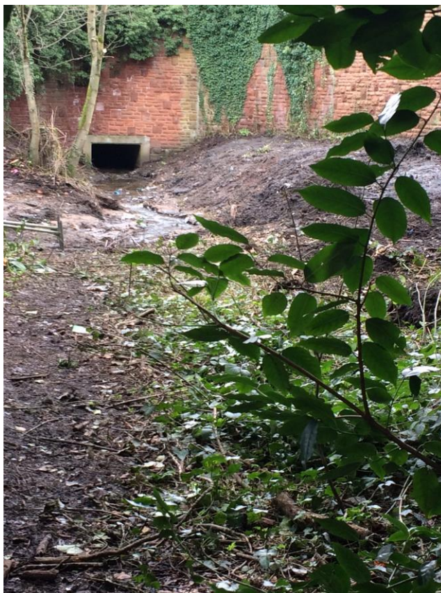
Figure 19: Top retention pond during clearance works
