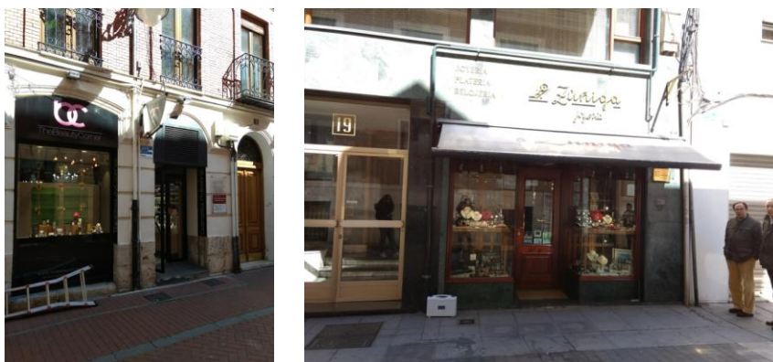
Figure 2.6: Temperature and relative humidity sensors installed in Santa María St (Source: CARTIF)
