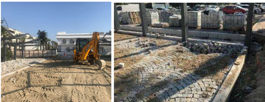
Figure 2-17: Sub-layer applications on Vilayetler Evi Car Park
