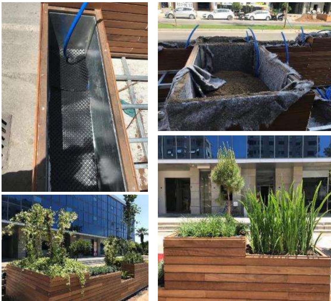
Figure 2-8: Activation of drip irrigation and planting the plant species
