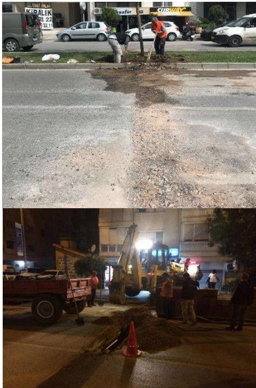
Figure 2-3: Connection of pipeline to parklets for drip irrigation
