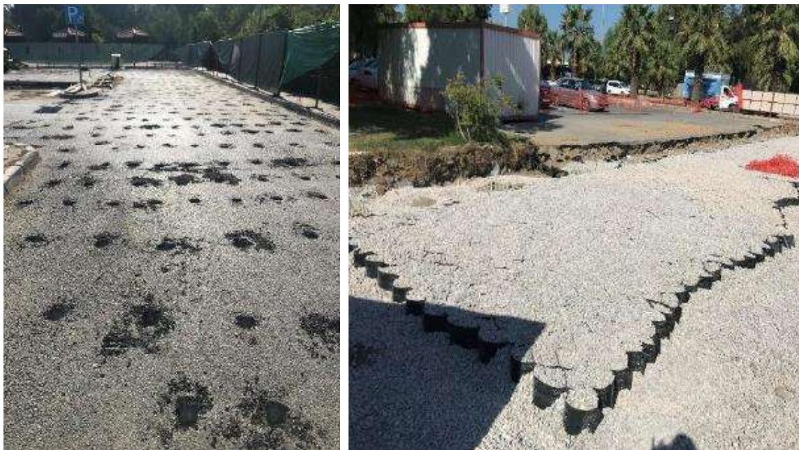
Figure 2-14: Removal of the existing surface and laying the layers of permeable surface
