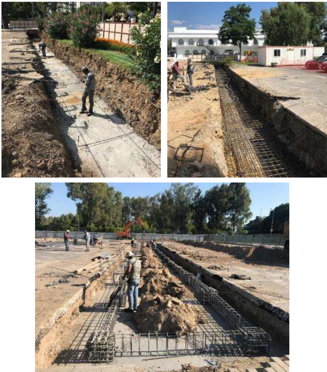
Figure 2-13 Construction work on green covering shelter foundation
