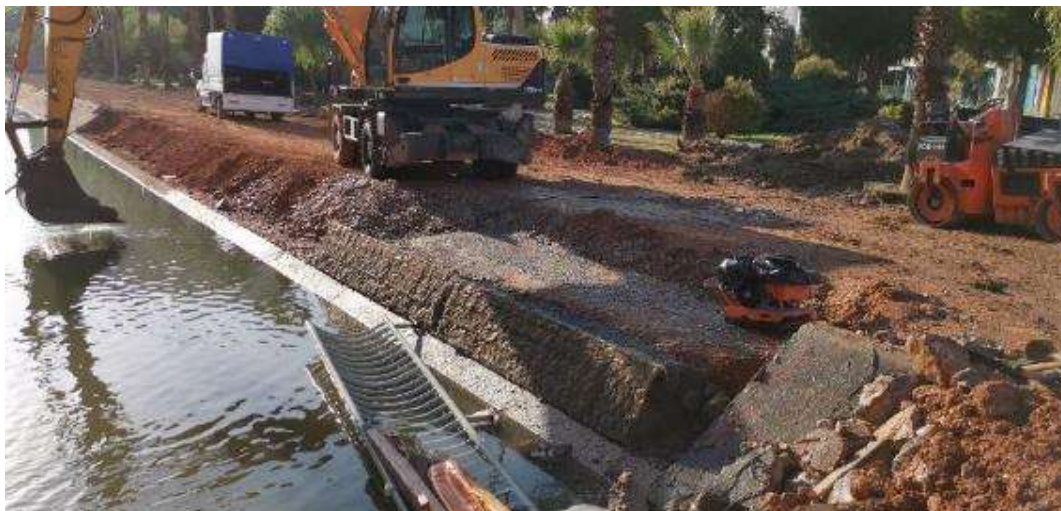
Figure 4-9: Sample terramesh application on the edges of the stream
