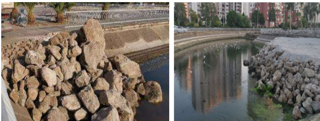
Figure 4-3: Stone filling application inside the stream
