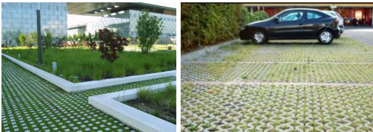
Figure 2-11: Examples of permeable pavements 3,4
