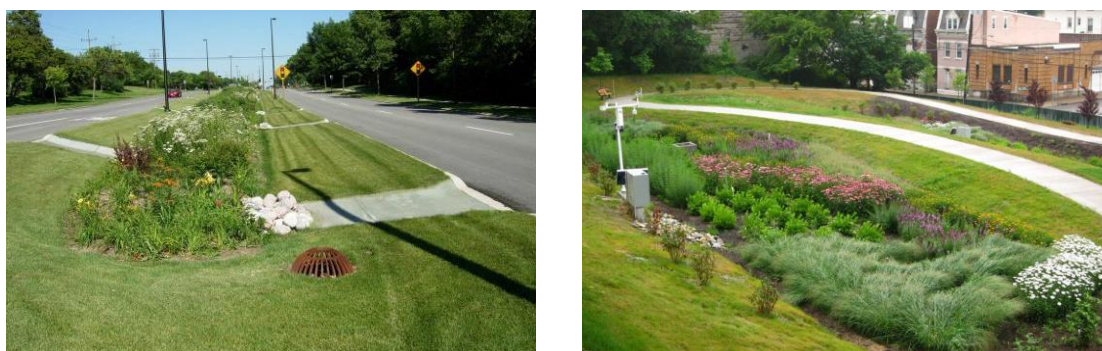
Figure 2.42: Examples of SUDs for rain water retention & infiltration: green swales and rains gardens
