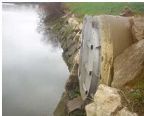
Figure 4.54: Detail of a non-return valve
