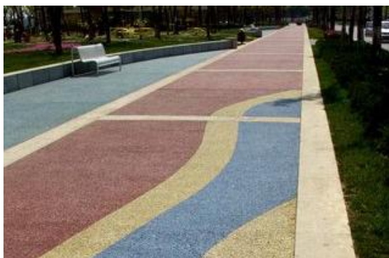
Figure 2.17: Pervious concrete cycle track (Source: www.perviousproducts.com )
