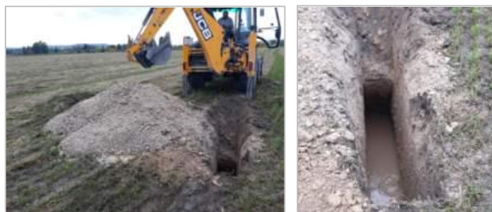
Figure 4.47: Excavator machine used to dig the pits and take out the terrain for its study
