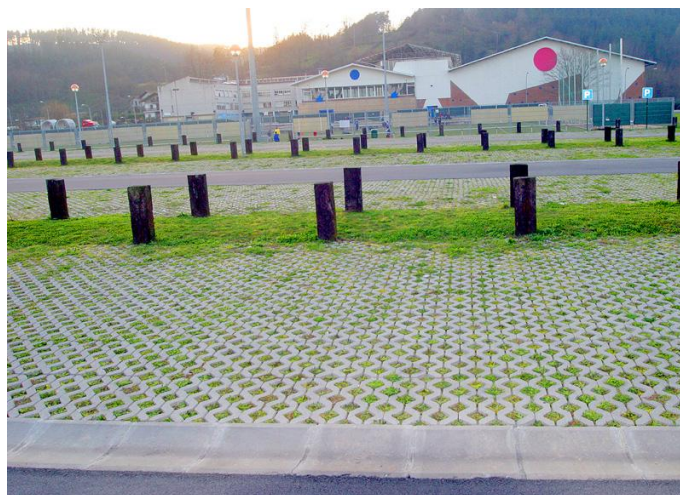
Figure 4.7: Example of a green parking area with prefabricated concrete blocks (Source: Alberdi 12 )
