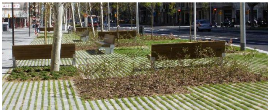
Figure 2.43: Examples of SUDS for rain water retention and infiltration: green pavements
