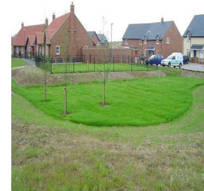
Figure 8 Detention basin – near play area
