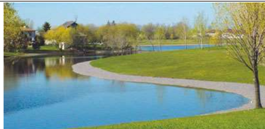
Figure 11 Stormwater retention pond
